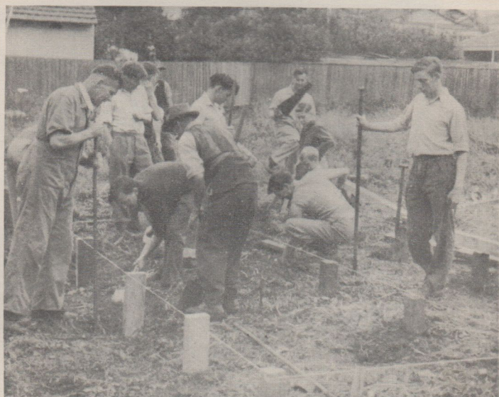
Putting in stumps for Masonite Hut.
